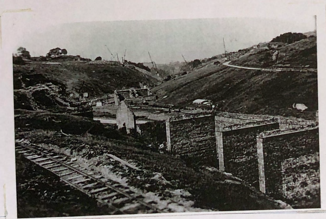
Remains of suspension bridge, Tacoma Res. construction
