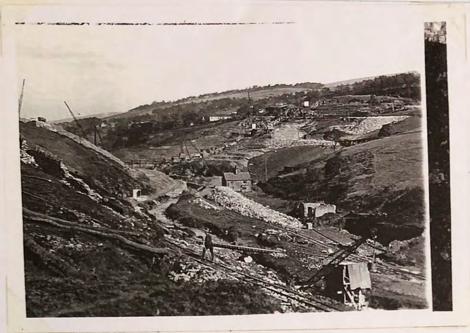
Construction of Fernilee Reservoir, early 1930's Cottages in middle of photograph were known as (Powder Mill Cottages.)
