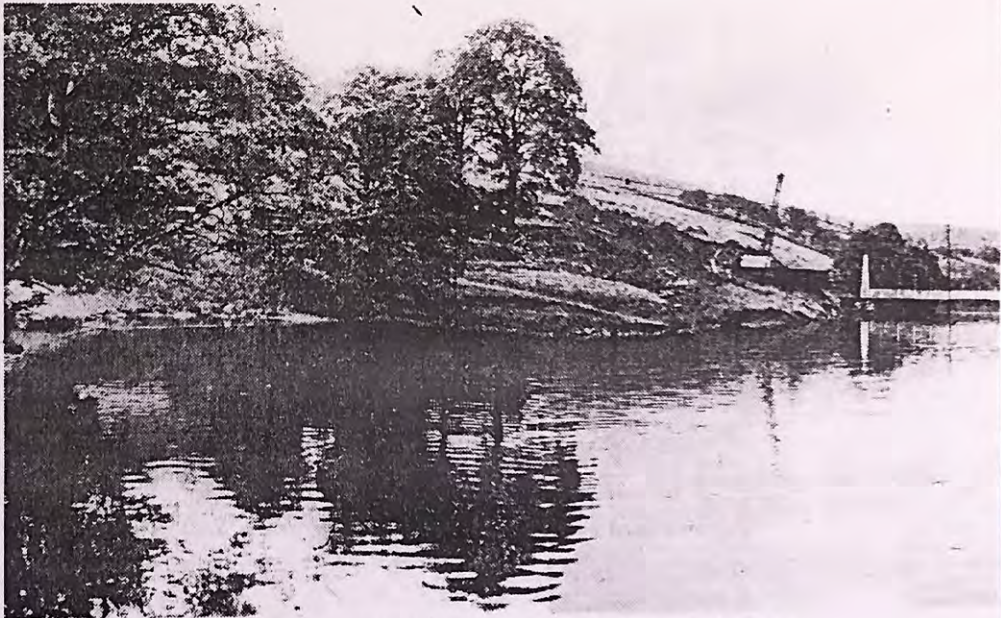
☆ The new reservoir at the Goyt Valley will be separate from the Fernilee reservoir but very close to it. The dam wall will rise from a point just beyond the bridge. This picture was taken from the Fernilee reservoir. A coffer dam is to be built this side of the bridge.
