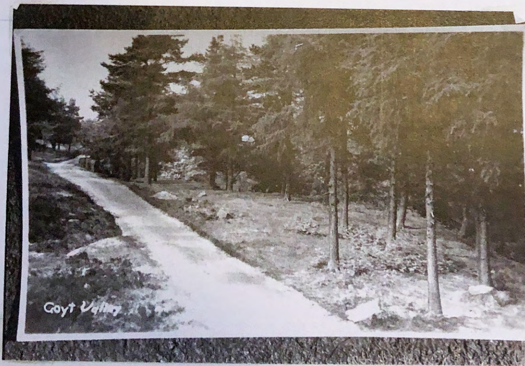
Coys Valley. Mid distance left is Stake Clough culvert wall on roadside
