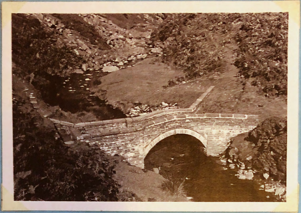
THE REBUILT PACKHORSE BRIDGE AT GOYTSCLOUGH.
