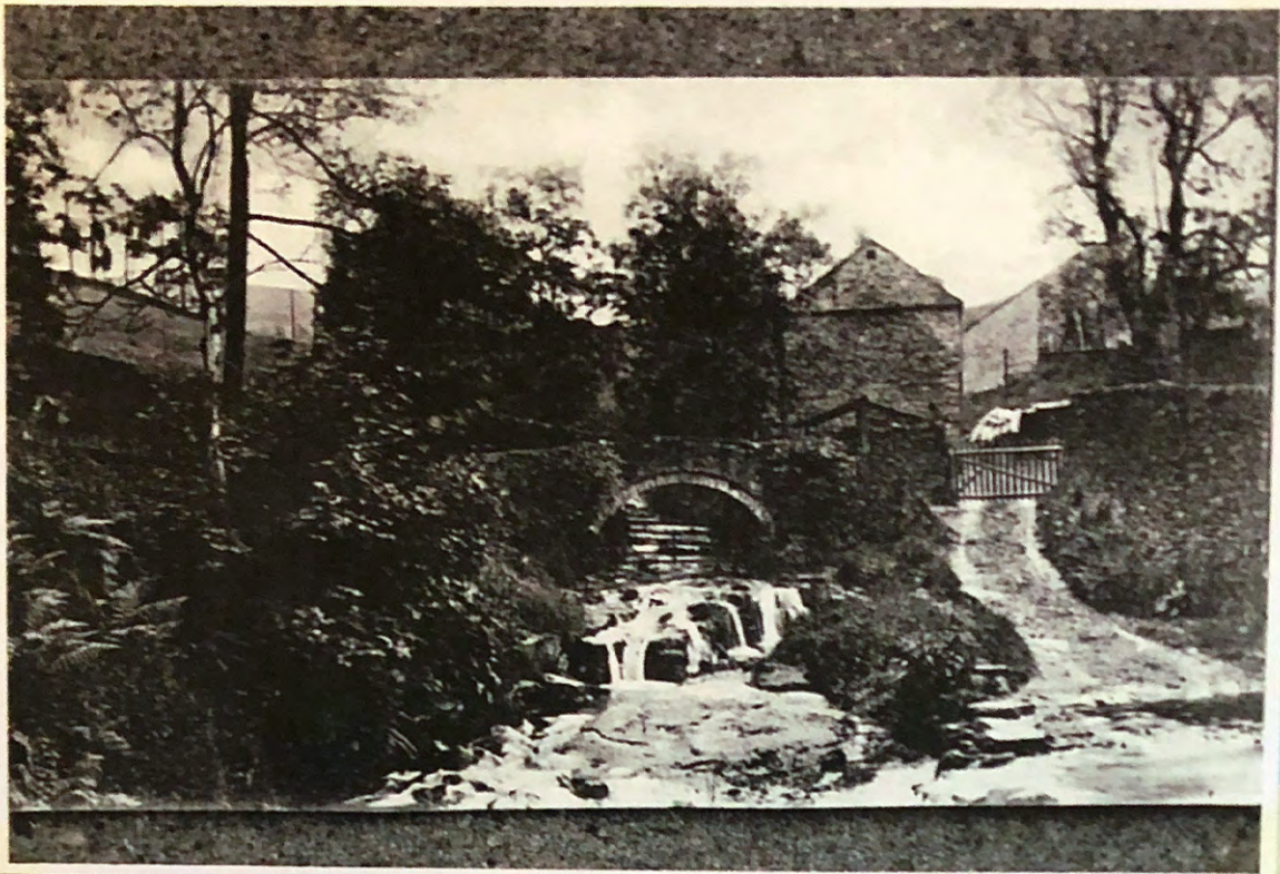
THE ORIGINAL PACKHORSE BRIDGE NEAR GOYTS HEAD BRIDGE FARM
