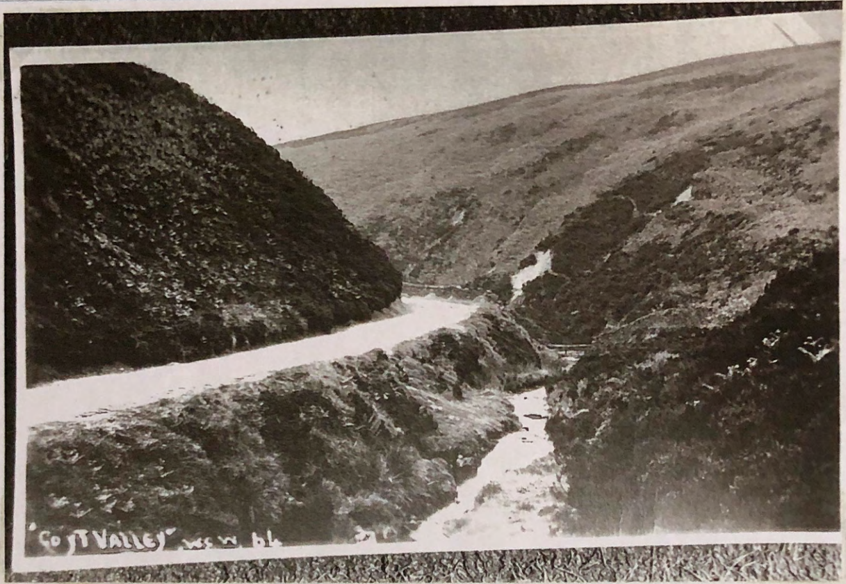
DOWNSTREAM OF LINDSAY BRIDGE (NOTE WALL TO SEVERAL CROSSING IN BACKGROUND)
