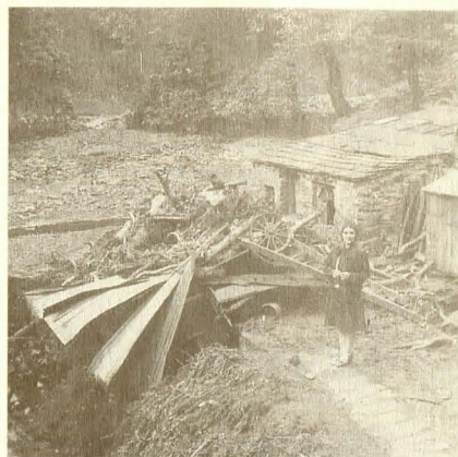
The Smithy, near the mine damage caused by flash flood, 1930.
