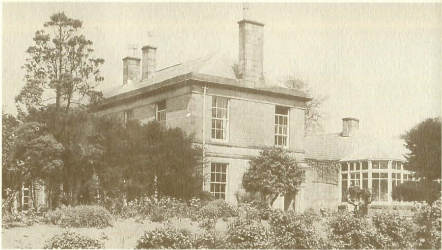
Ingersley Hall, home of the Gaskell family.
