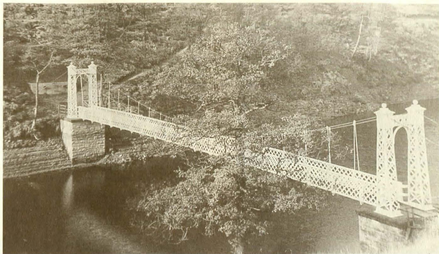
This pretty suspension bridge was removed for the construction of Errwood Reservoir.
