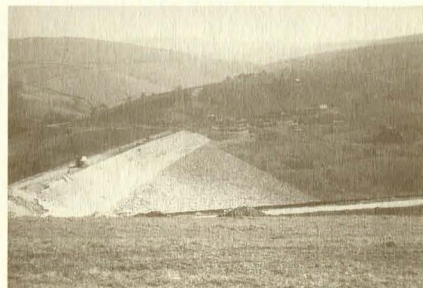
Errwood Dam nearing completion.
