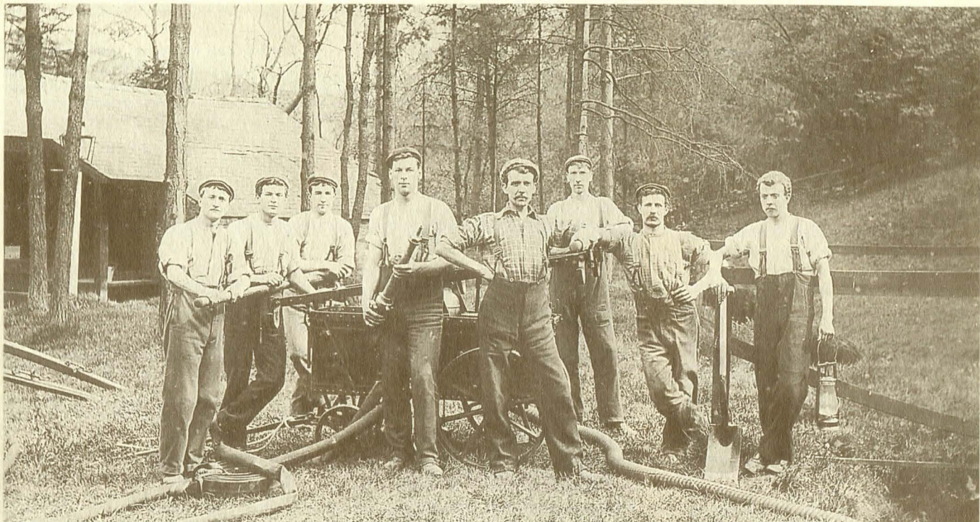
'Fire Fighters' of the Gunpowder Works.
