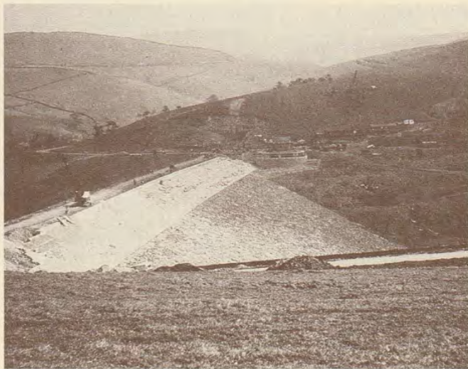
Errwood Dam nearing completion.
