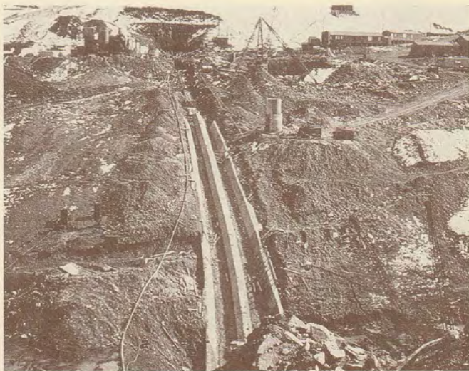
The trench for Errwood Dam wall.
