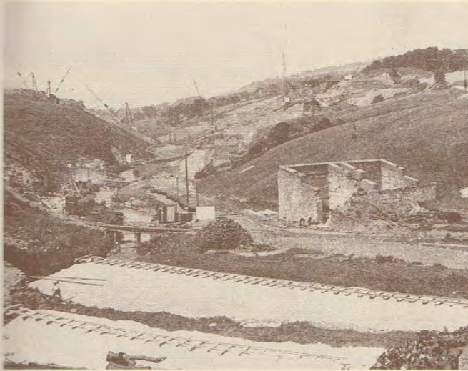
Construction begins on Fernilee Dam.
