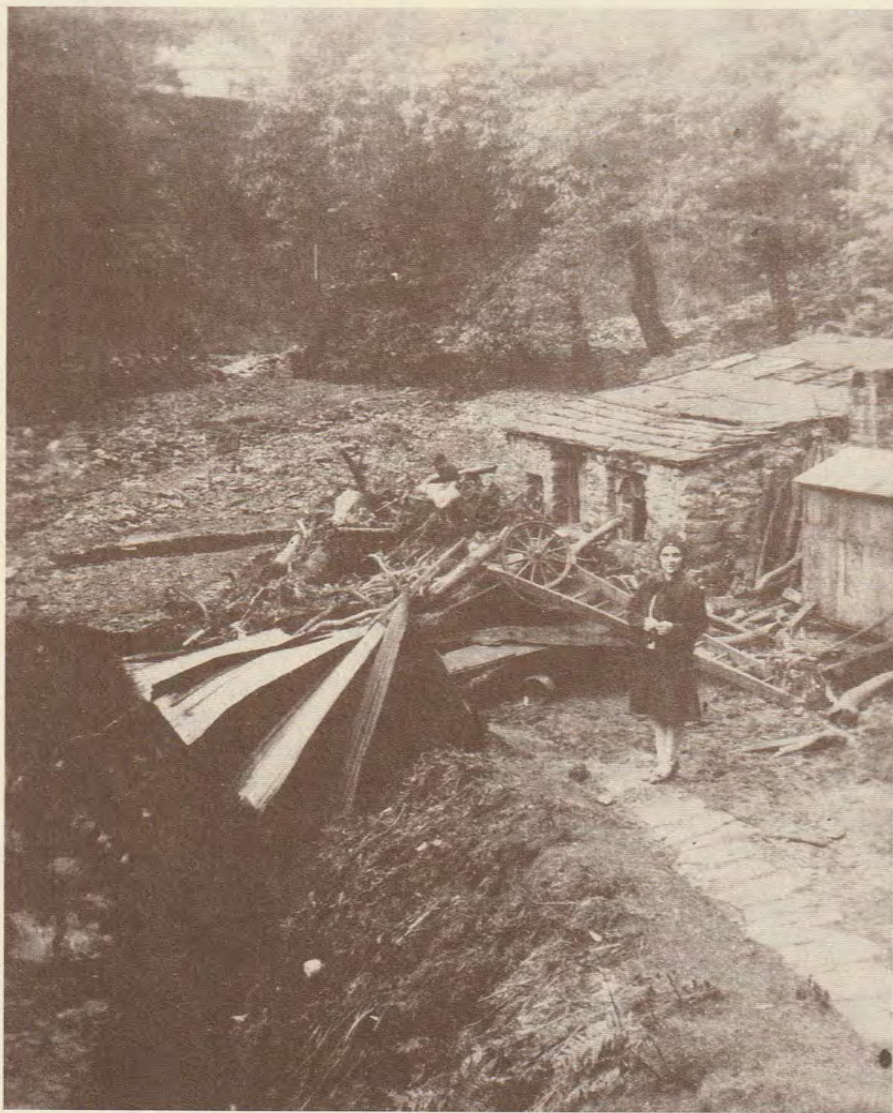
This was the Smithy near the mine. The damage was caused by the flash flood in 1930. They had a circular saw here for making pit props.
