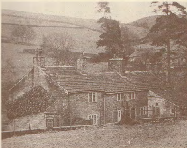
View from the rear of the Gatehouse Cottage.
